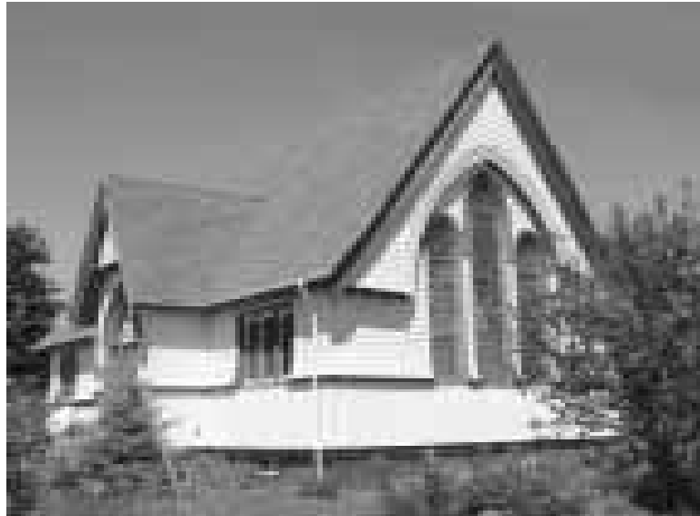
Londonderry Church is one of the historically significant churches to be documented in an historic places project.
