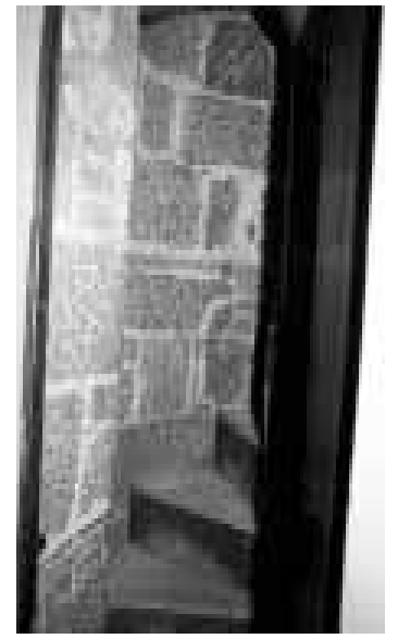
The stairway to the bell tower was a tight squeeze for firefighters.
